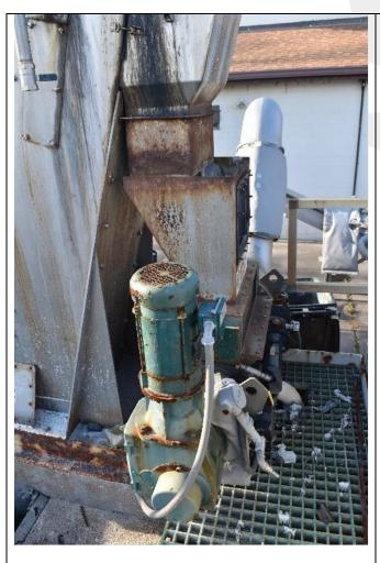
needs to be removed to ensure proper operation. Note the amount of corrosion at the influent structure while in open-air conditions. This is an indication of septic conditions and high hydrogen sulfide concentrations.
